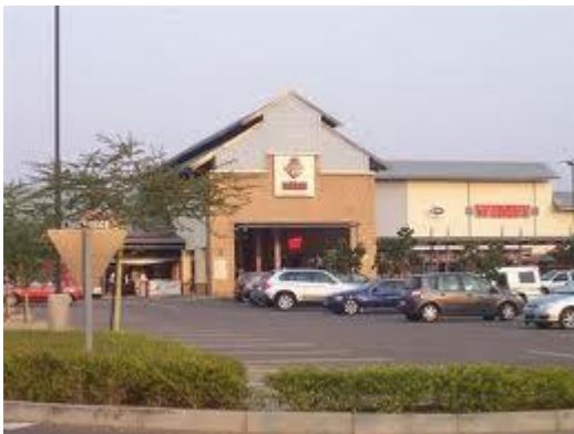
Picture 2-1 Makhado Crossing Shopping Centre
