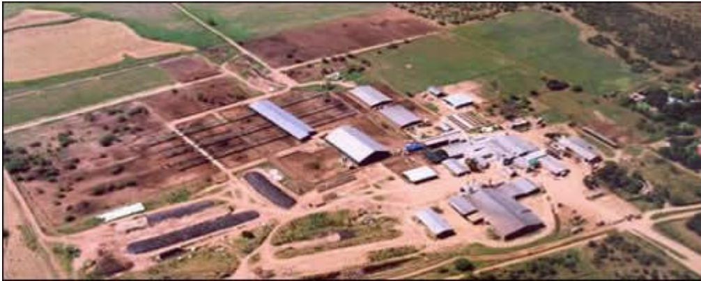
Picture 3-3 Limpopo Dairy Processing Plant
